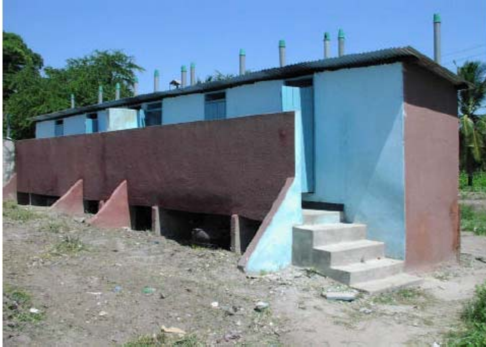
Figure 5: Ecosan toilet at Karakata Primary School in Dar es Salaam
