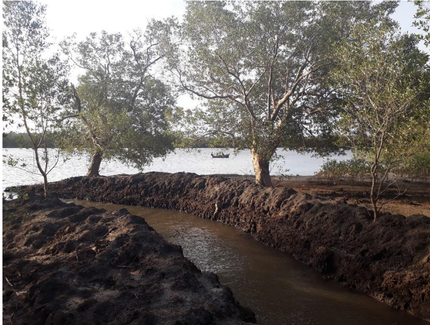
Figure 4. The entrance (from the estuary) to a hand-dug channel leading water to barren areas identified for hydrological restoration.
