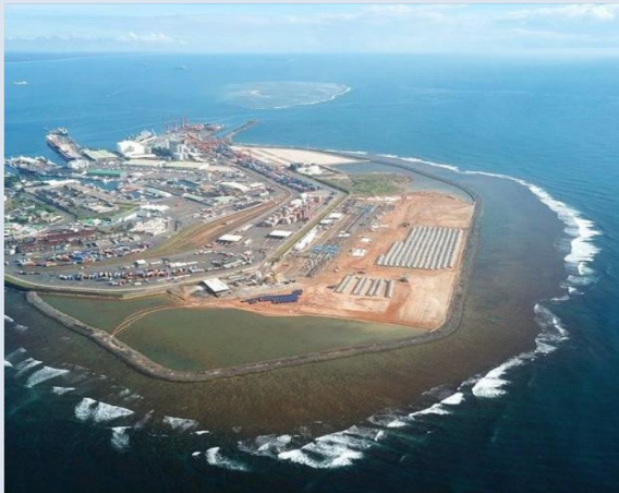
View of expansions in the Port of Toamasina
