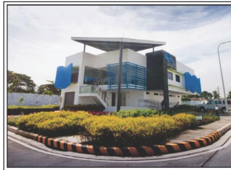
East La Mesa Water Treatment Plant
