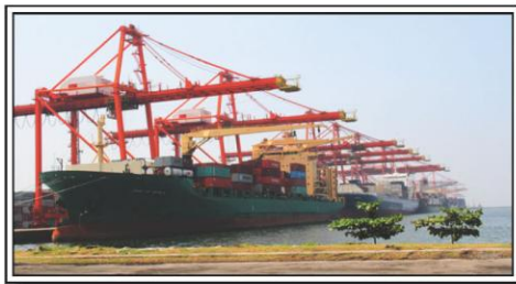
International Container Terminal Services, Inc.
