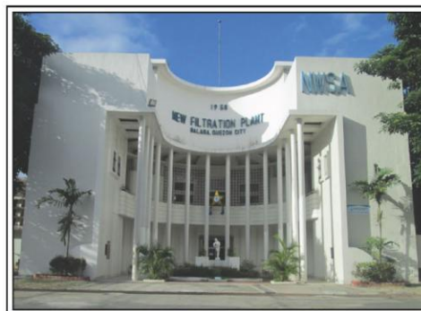
Balara Water Treatment Plant
