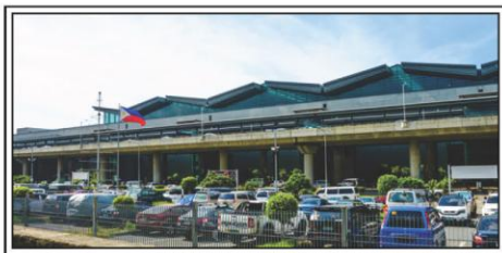
Ninoy Aquino International Airport
