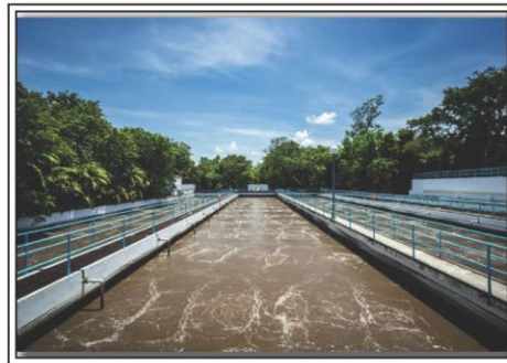
Maynilad's Alabang Sewage Treatment Plant
