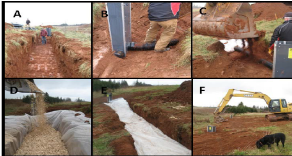
Figure 4.9 Bioreactor construction steps: “(A) trench construction, (B) flow control structures, (C) backfill pipes and control structures, (D and E) placing plastic liner and filling trench with woodchips, (F) final soil coverage” (Source: http://www.knwsa.com/pdfs/Bioreactor_20140210.pdf )
