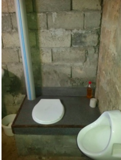
Figure 5: Construction of demonstration objects like UDDT toilet in Khorga
