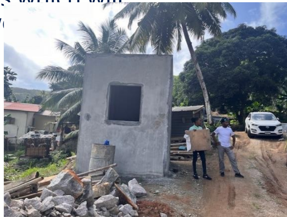
Generator and pump room
