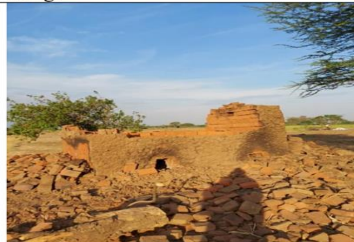
Brick laying along Mbarali river at Mwakaganga area- Ubaruku
