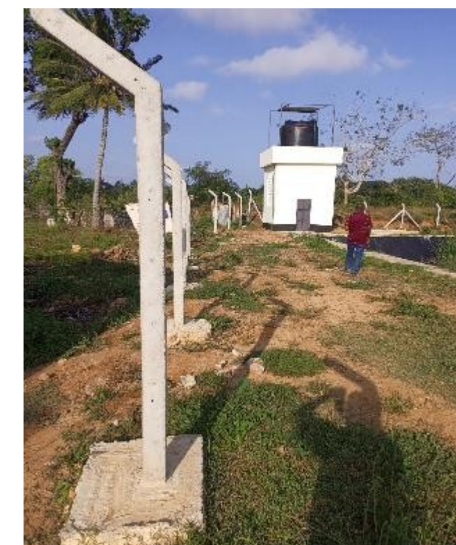
4. Water tower equipped with tank-fenced site
