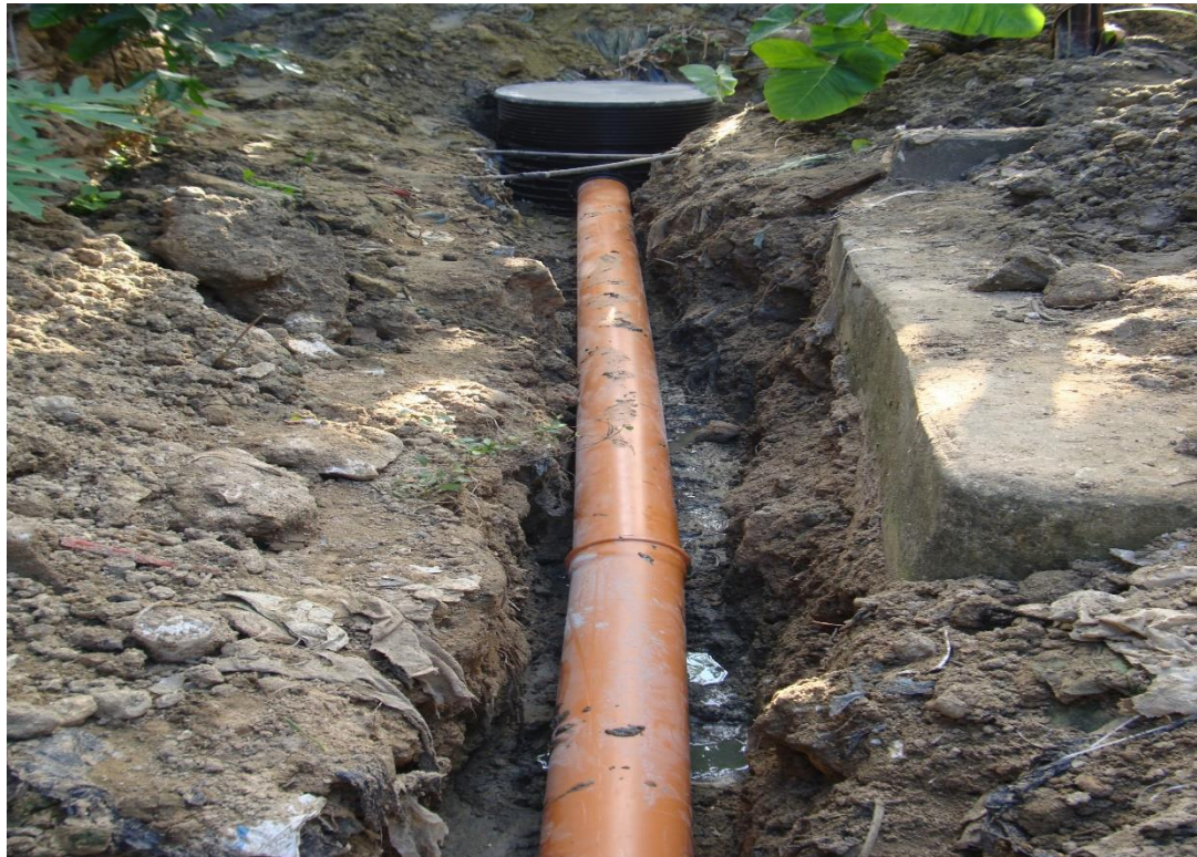
SEWAGE LINES UNDER ALIGNMENT
