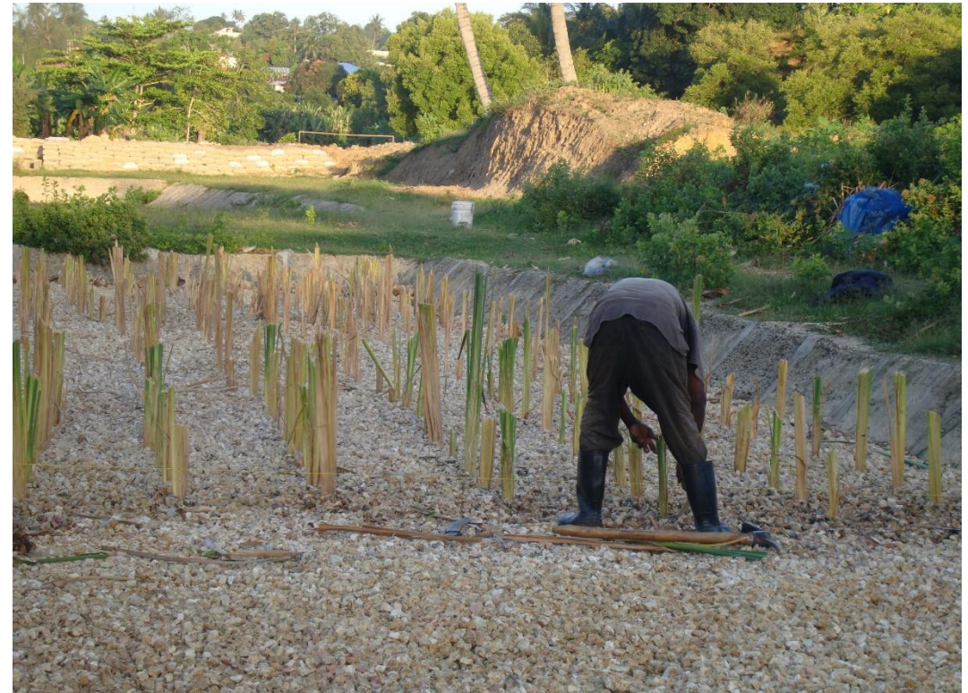
COMPLETING THE WETLAND POND
