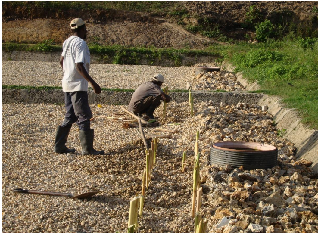
CONSTRUCTION WORKERS IN ACTION
