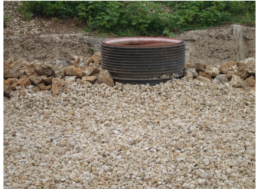
LAYING INLET LINES INTO THE PONDS
