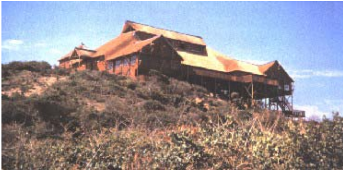
Plate 1. A tourism infrastructure built in a coastal dune. The project was approved by the municipality, but it did not have the approval of the Ministry of Environment.
