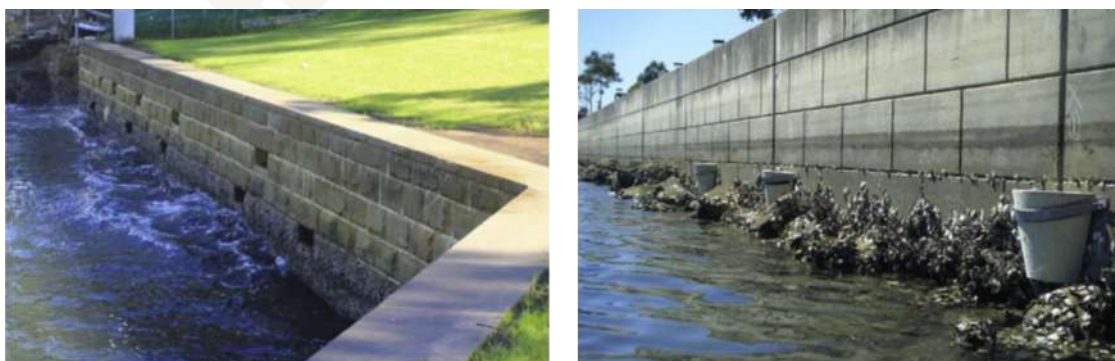
Figure C.7 Example of cavity pools (left) and flowerpots (right) on vertical seawalls (source: Morris et al. 2018)
