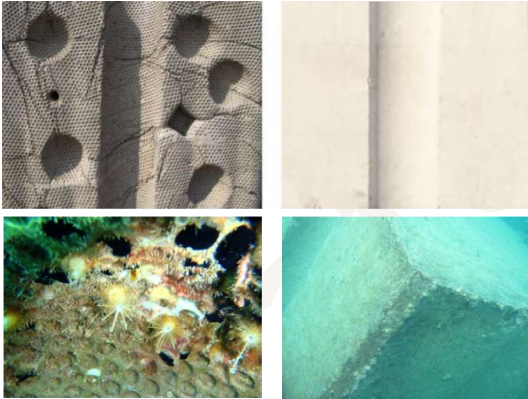
Figure C.6 Example of ecologically enhanced armouring units (left) and standard units (right), also showing colonisation over similar periods (source: Ido and Perkol-Finkel 2015)
