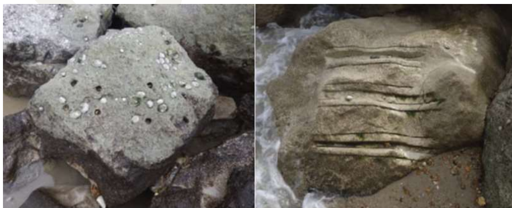
Figure C.5 Example of artificial microhabitats (holes and grooves) on boulders to mimic natural microhabitats (source: Hall et al. 2018)
