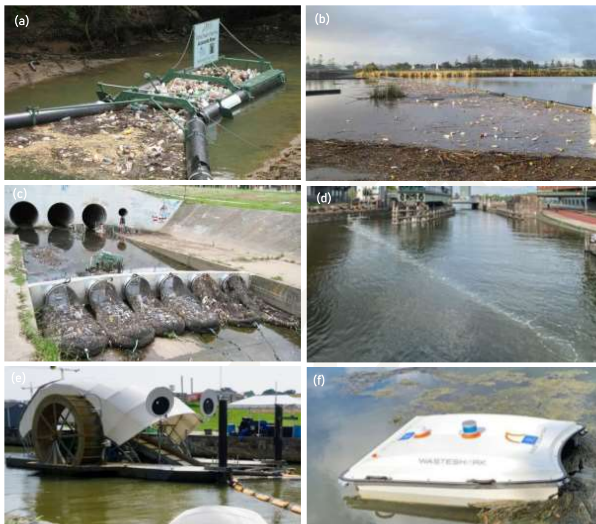
Figure E.13 Examples of a (a) litter trap, (b) litter boom, (c) net trap, (d) barrier (e) litter skimmer and (f) aquatic vacuum (Sources: see Table E.17)
